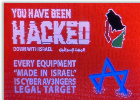
Altered image threat actors placed on water utility monitoring devices
